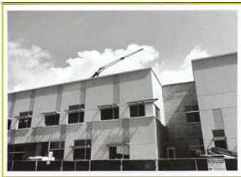
Main Library Construction, Mar 2005
